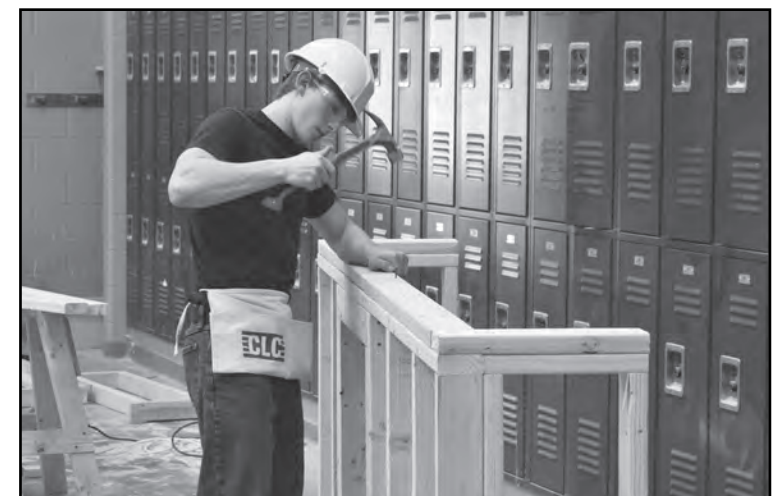
AUSTIN MARTIN BUILDS THE WINNING WALL. PHOTOS BY LIAM PARIDO
